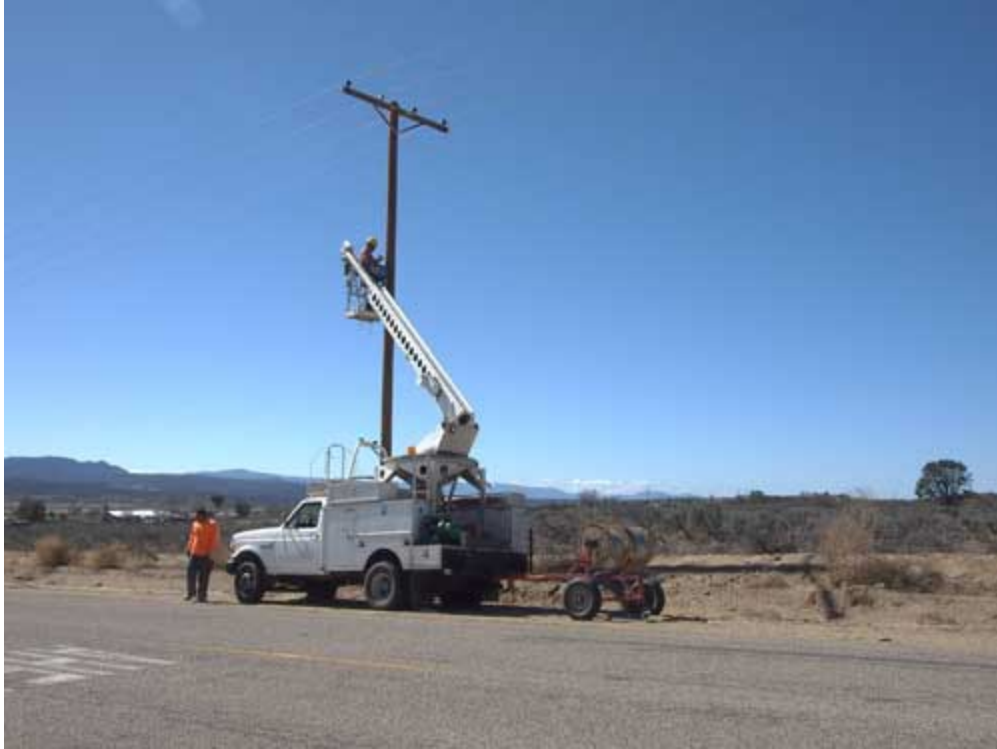
Installing messenger wires on electrical utility poles for fiber installation.
