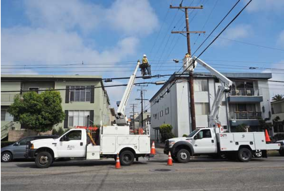
Two trucks lashing cable to a messenger. The lasher is just to the left of the pole.
